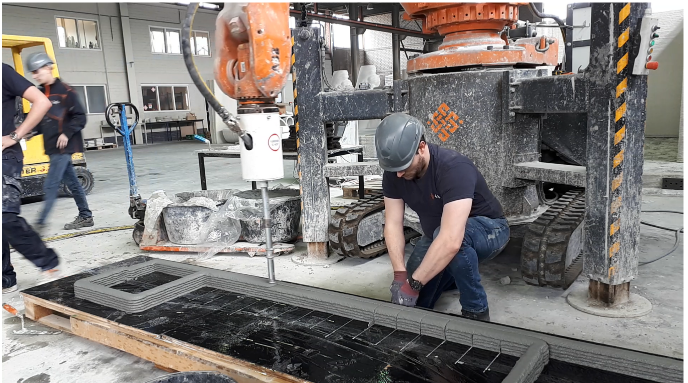
Fig. 9 Versarien's graphene utilised in a 3D printed mortar. Credit: CyBe Construction.
